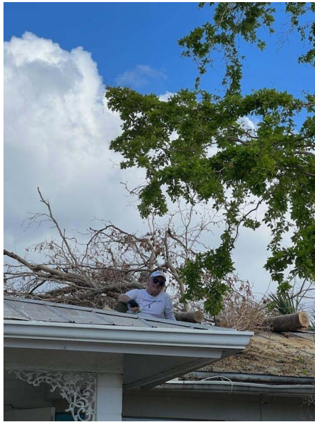
Linda Graves Arnold on bravely balancing on top of a home clearing tree limbs. Barb Ellis cleaning up tree debris safely from the ground. Bob Stern, "the man with the chainsaw" on top of the house in spite of his need for a knee replacement!
