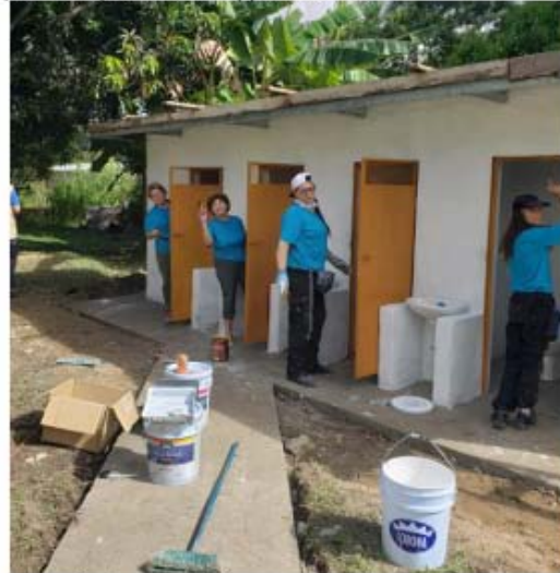
Our team working on school bathrooms.
