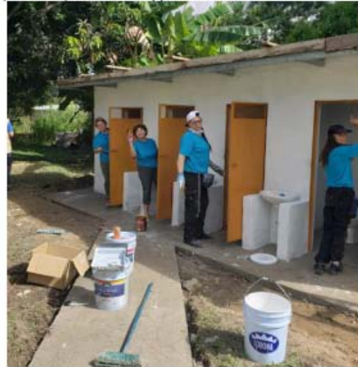
Our team working on school bathrooms.
