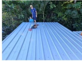
Mark Vernick & Gerry Cachia inspect roof repaired
