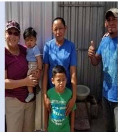
Installation of Latrine for family of 4 - Honduras 2022
