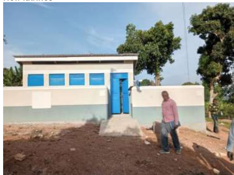
Fixing up classrooms
