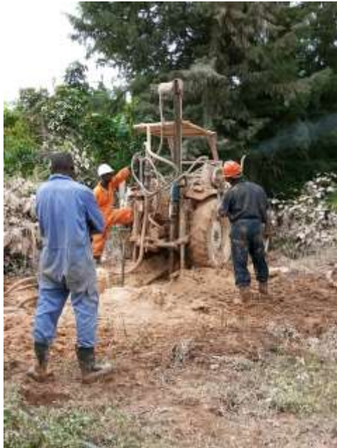
Boring for potable water already with our Global Grant (submitted by Stan Grogg)
