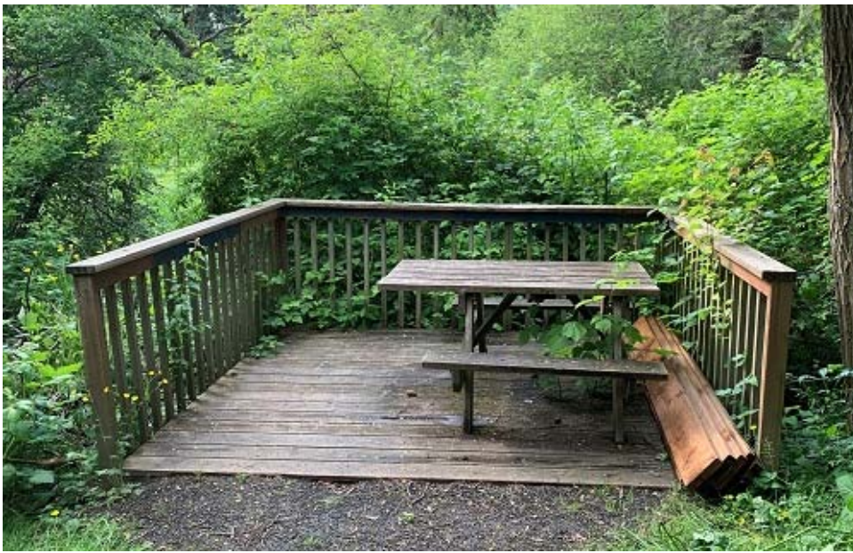
The "Before" photo of the platform on the Clear Creek Trail
