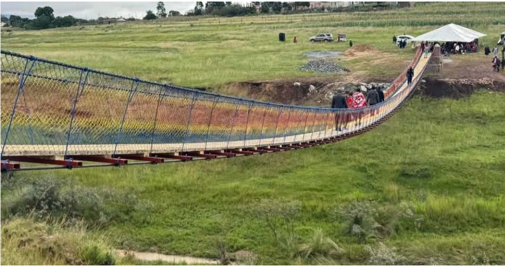
LAKHAYA FOOTBRIDGE MASEYISINI, ESWATINI MARCH 2025
