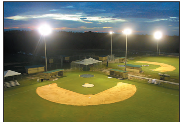
Francis Ball field after lights were installed.
