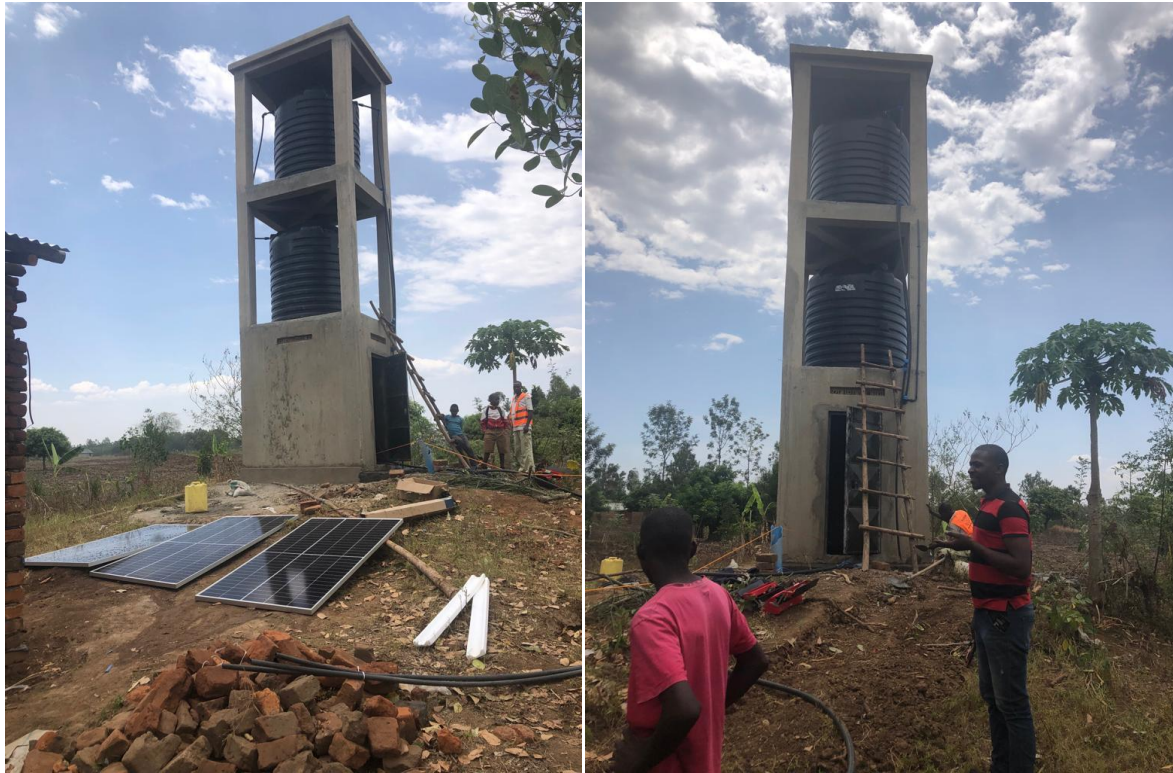
Water tower and pump house installation of water pump and solar systems at Kibumbire zone site.
