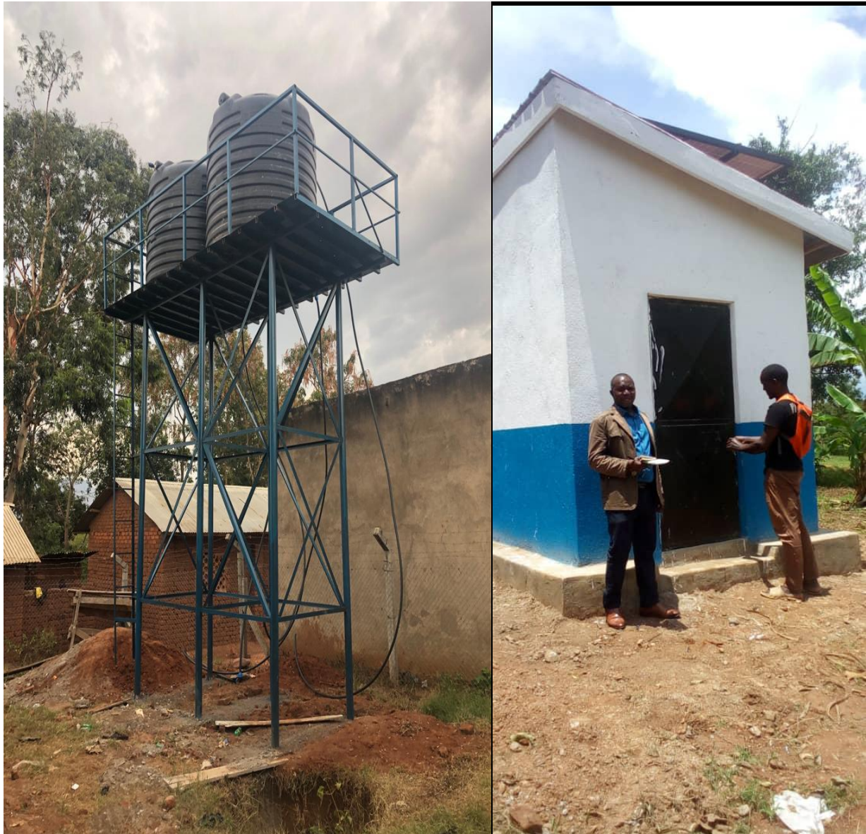
Water tower in Namabasa at Linda Good Samaritan p/s serving two kiosks at Namabasa III A site Fabricated and Pump house constructed at Namabasa zone III
