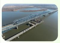
That original span was intended to carry five thousand vehicles a day, it now carries twenty-thousand vehicles, is well past its lifespan and will be replaced by the span under construction. That new span will be three lanes wide, as well as having a walking/bicycling lane. That new span is expected to last 70 to 80 years, although it will need resurfacing before it
