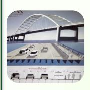
Here's a question: what has 74 thousand pounds of concrete, 21 miles of electrical cable, 40 million pounds of steel and 14 thousand tons of asphalt? The answer is the new east-bound span of the McClugage Bridge.
