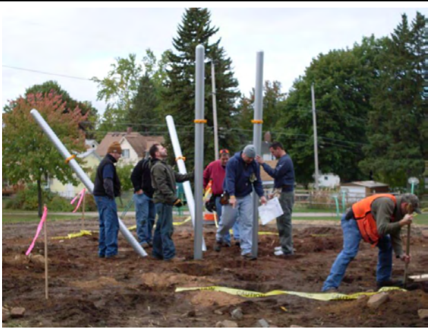
Putting in the main supports for the playground equipment
