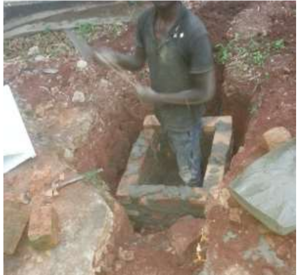
PREPARING WASTE WATER MANHOLE
