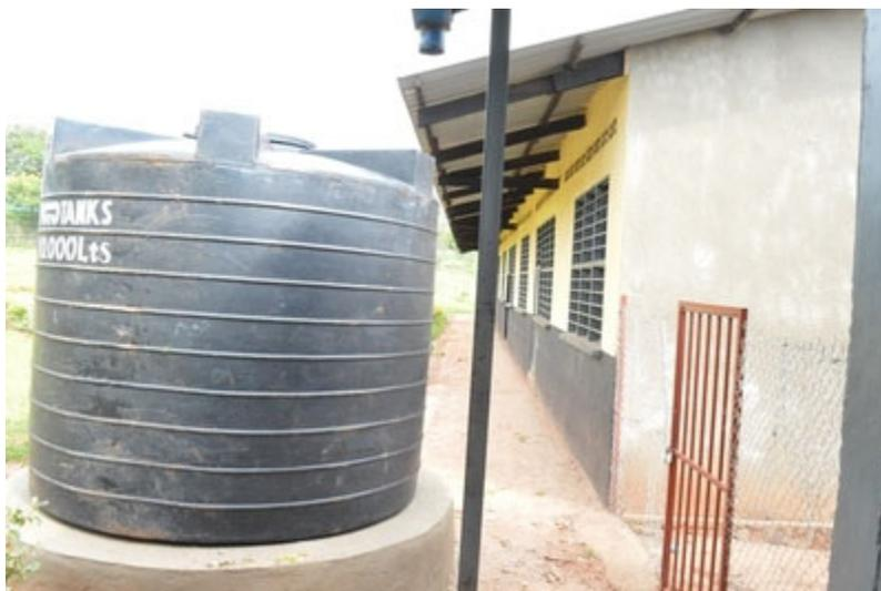
The water tank has been located on site. Two are being installed, Each are 10 cubic meters. Gutters and piping are being installed to catch rainwater and fill the tanks.
