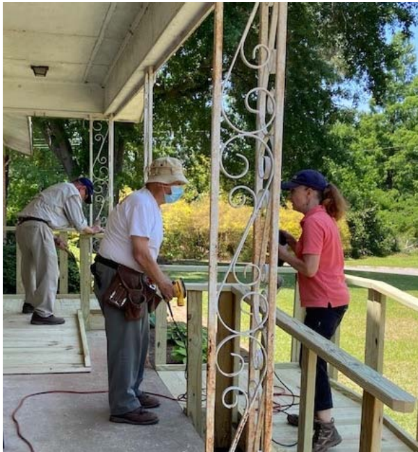
Thursday morning ramp builds with Resources for Seniors
